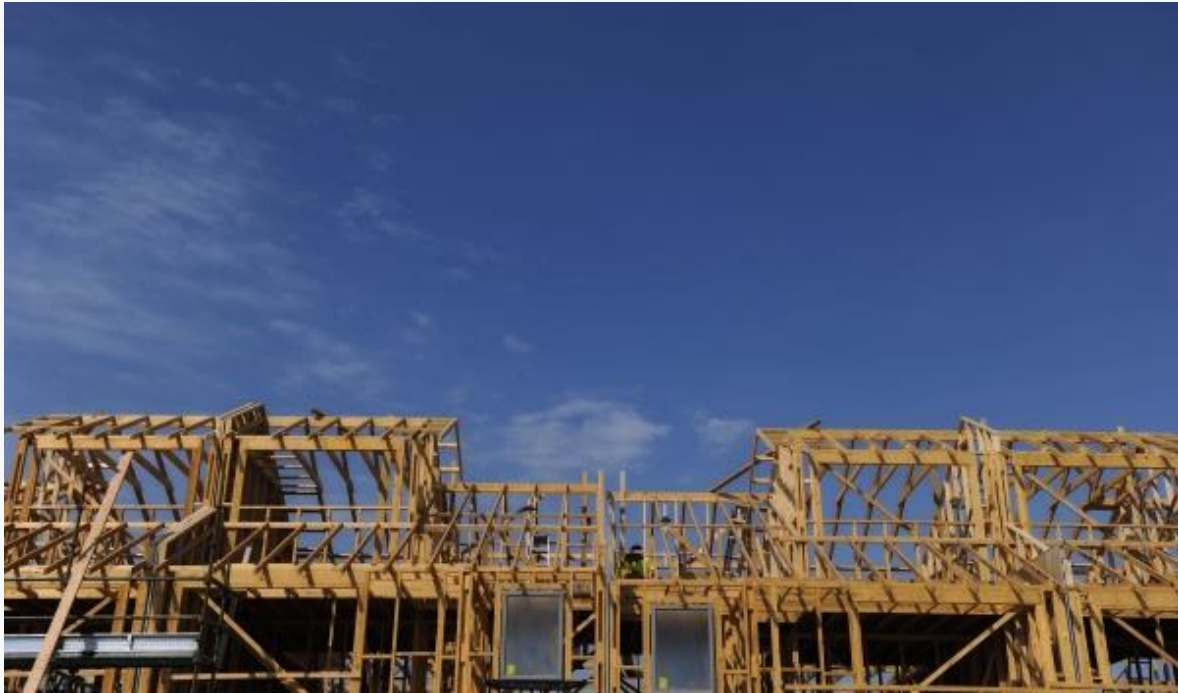
Timber frame for a new home in Western Sydney.
